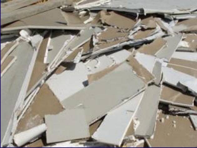
Gypsum wallboard waste
