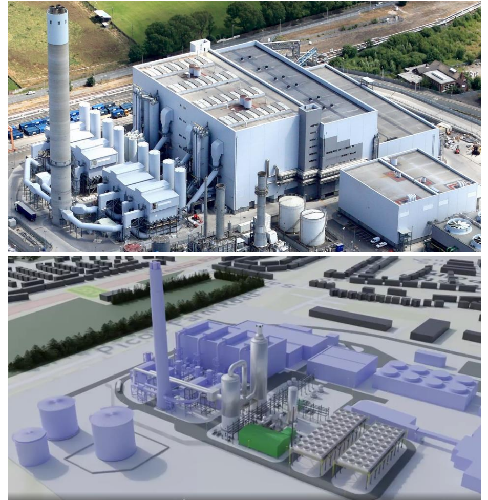
WtE plant combined with CC in Runcorn, UK
