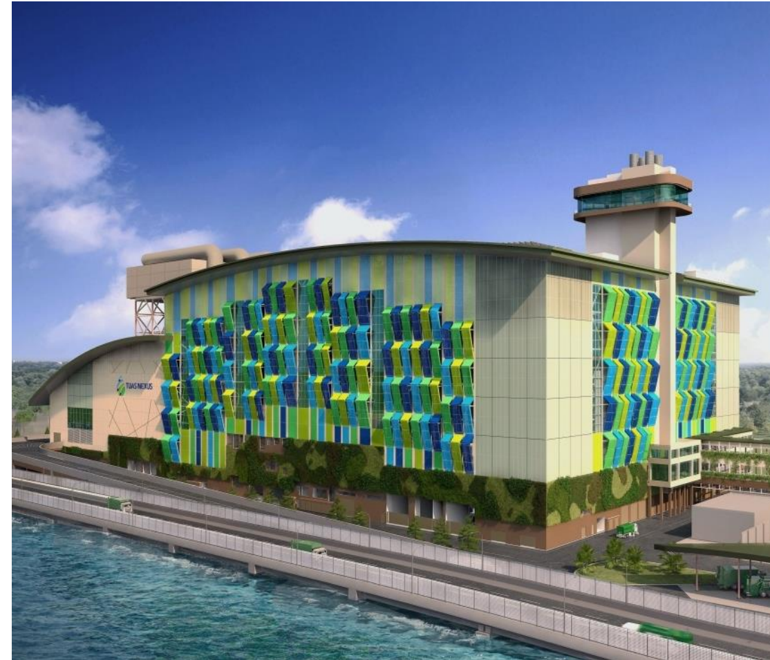
WtE plant in Singapore
